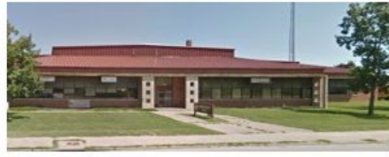
Central Office Burlington
